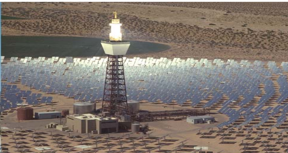
solar tower 塔式(SNL)
