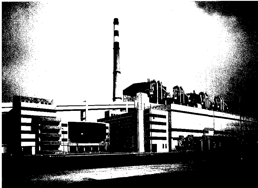
Qingdao Thermal Power Plant (2 × 300 MW)—one of the six pilot units for “separating power plants from networks and bidding for access to networks”
