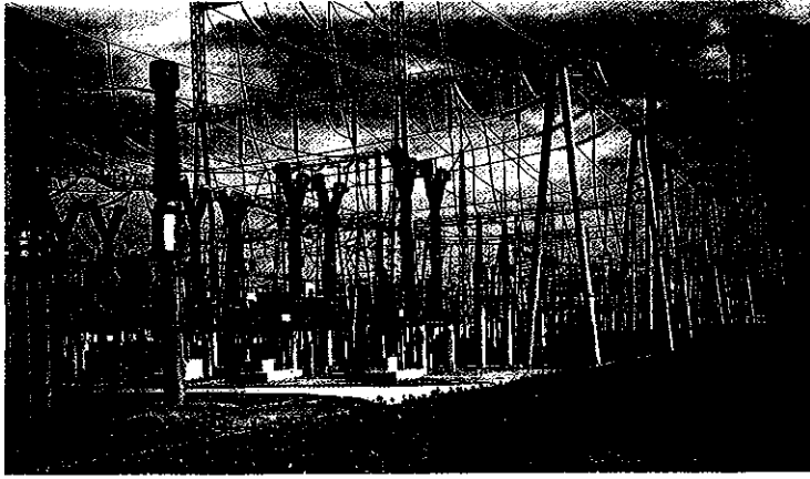
Jining Maqing Substation, Shandong
