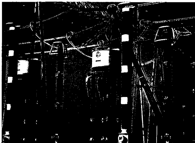
Installation of the outdoor electric equipment for Three Gorges-Wanzhou 500 kV Substation, Sichuan
