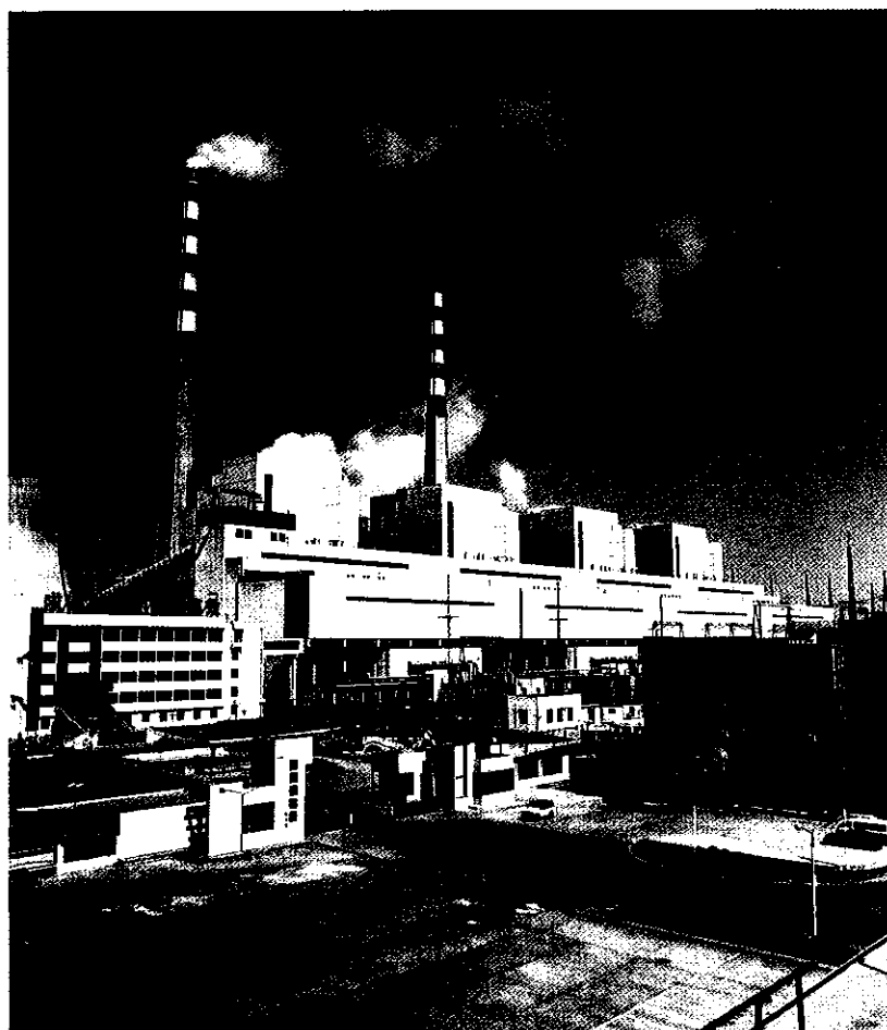
Tieling Power Plant (4 × 300 MW), Liaoning
