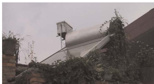
FIGURE 8 Flat-panel solar water heater, Yunnan province.
