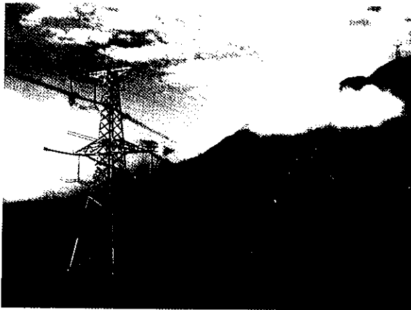
Zigong No.1 500 kV transmission line
