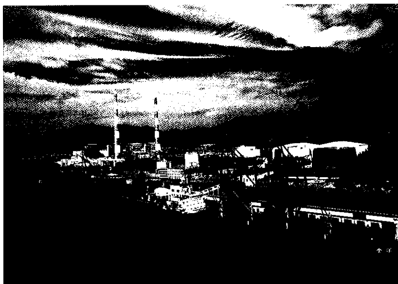
Huaneng Fuzhou Power Plant along Minjiang River
