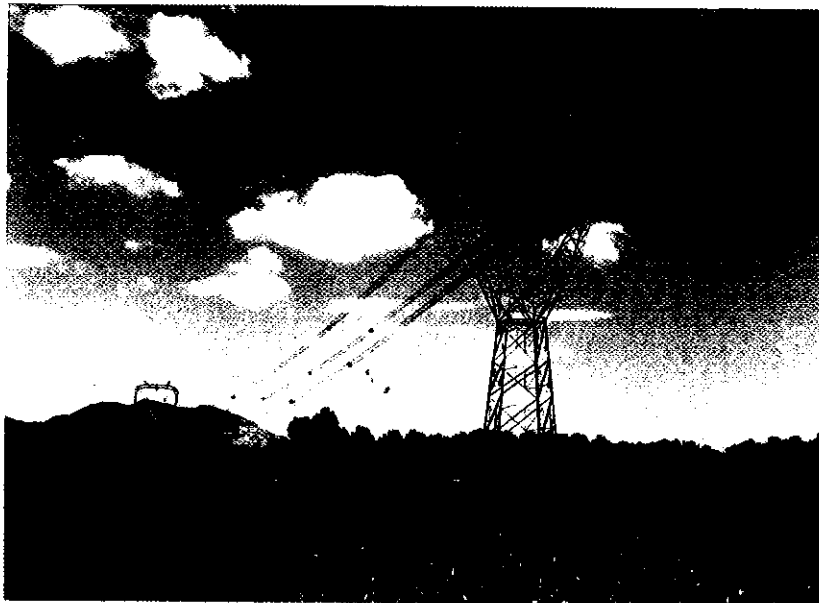
The 500-kV compacted transmission line from Changping to Fangshan
