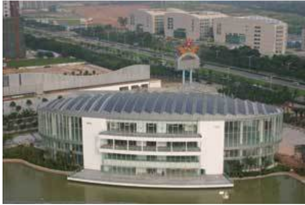
Building integrated photovoltaics on a new building in Shenzhen WANG SICHENG, BEIJING JIKE NEW TECHNOLOGY CO
