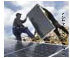
image BERLINER GEOSOL INSTALLING THE SOLAR ENERGY PLANT (PHOTOVOLTAIK) "LEIPZIGER LAND" OWNED BY SHELL SOLAR IN A FORMER BROWN COAL AREA NEAR LEIPZIG, SACHSEN, GERMANY.
