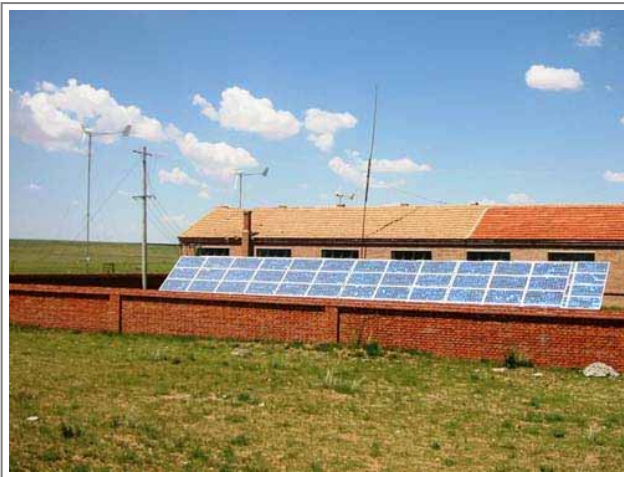
14kW solar PV array and 20kW of small wind turbines are part of a wind/solar/diesel hybrid off grid power supply for a village 200km northeast of Hohhot, Inner Mongolia. Photo - 2004
