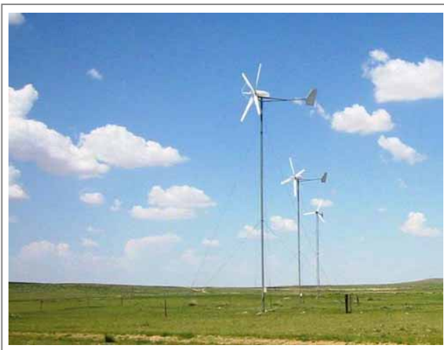
Three 10kW wind turbines supplying power to an off grid village in Inner Mongolia. Photo - 2004
