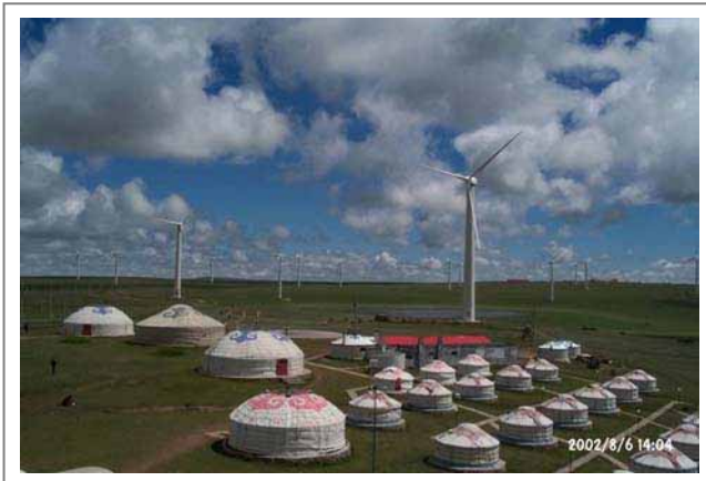
Grid connected wind farm in Inner Mongolia. Photo - 2002
