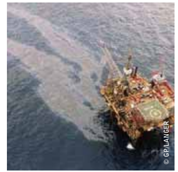
image PLATFORM/OIL RIG DUNLIN A IN THE NORTH SEA SHOWING OIL POLLUTION.
