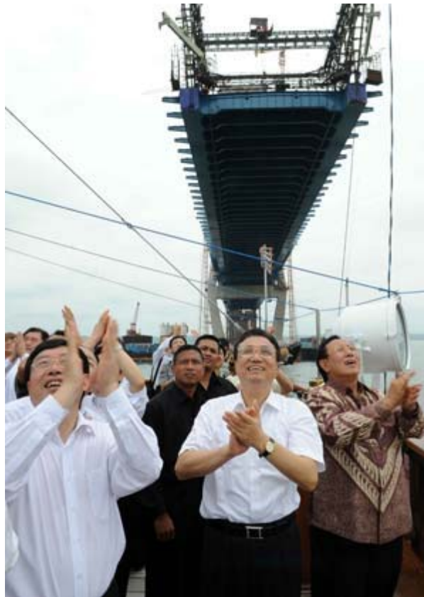
Visiting Chinese Vice Premier Li Keqiang (C front) applauds as he visits the construction site of the Suramadu ( Surabaya-Madura) bridge, which will be the longest of its kind, in Indonesia, Dec. 21, 2008. (Xinhua Photo)
