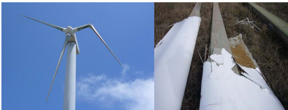
Damaged V42 blade
