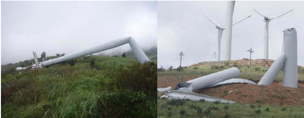
Broken wind turbine tower frame
